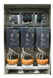
QULON-D is smart supplement solution to stabilize and control voltage in three-phase networks with conventional lamps. Only by providing phase dimming in 180-245V range for 230V networks QULON-D saves up to 40% of energy costs and prolongs lamp lifetime (due to "soft start"). Dimming module provides wide range of diagnostic tools of output power lines as well as incorporates overload protection and short circuit resistance including built-in automatic bypass.
